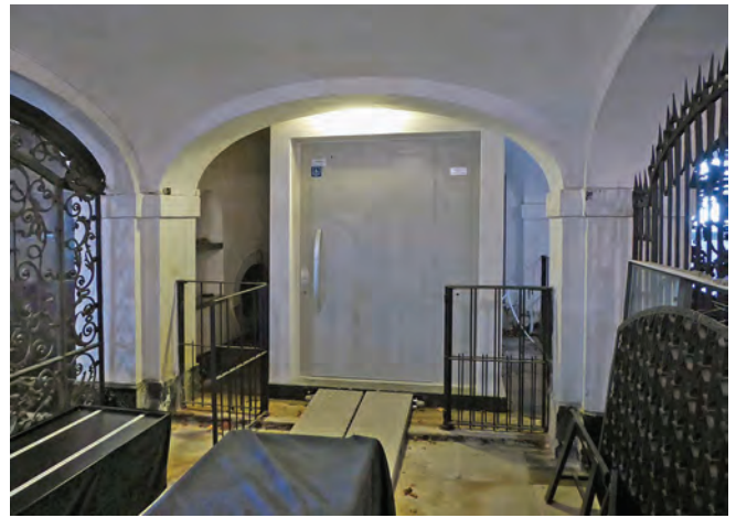
The Coffin Lift beneath Christian's Church is an unusual addition to the crypt which was consecrated in 1759. The ramp and covered bier can be seen leading out of the lift doors. Photo Martin Dixon
